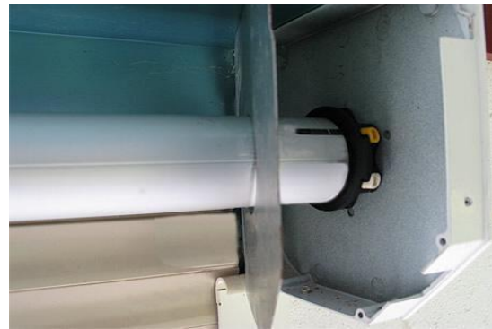
electric motor on right side of roller shutter.
